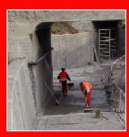
Alternatively apply VANDEX SUPER as a slurry.
