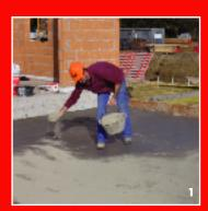
VANDEX SUPER dry-sprinkled as powder immediately after initial setting of concrete.
