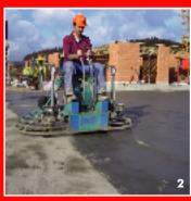
Working the powder into the surface by machine or hand trowel.
