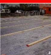
Curing and protection for 5 days against evaporation by sun and wind.
