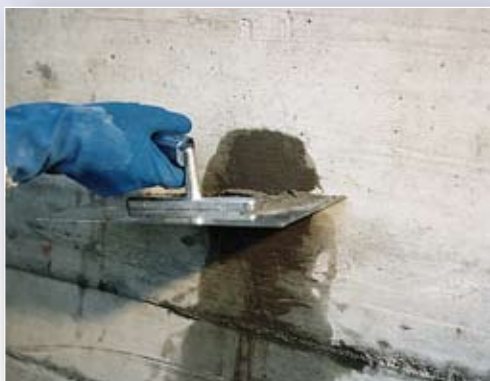
Level off surface.
