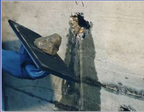
VANDEX PLUG fresh mortar ...
