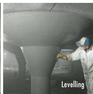
Spraying levelling mortar
