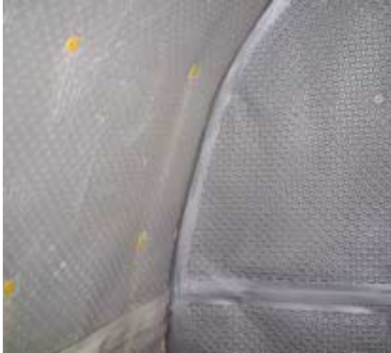
4. The membrane is secured using the special Oldroyd Brick Plug and compression seal.
