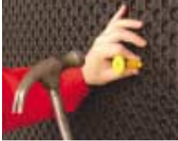
4. The membrane is secured using the special Oldroyd Brick Plug and compression seal.
