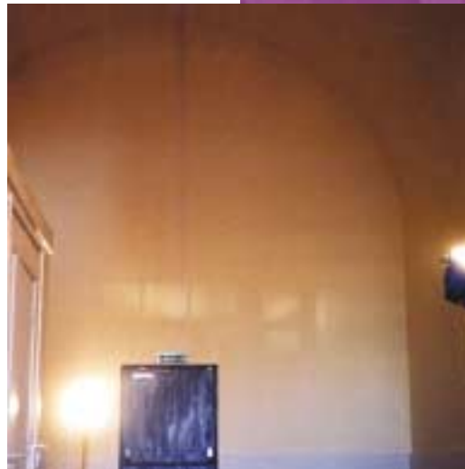
Finished rendered surface
