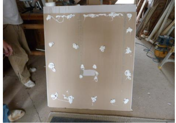
Drygrip dabs applied to plasterboard.
