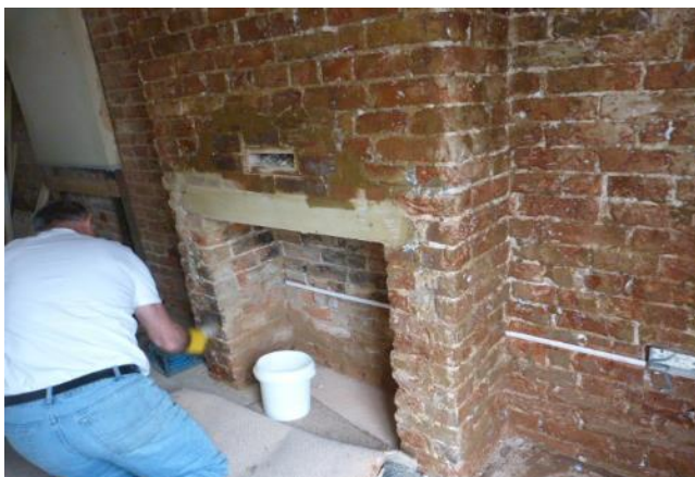
Dryshield applied to fireplace outer walls.
