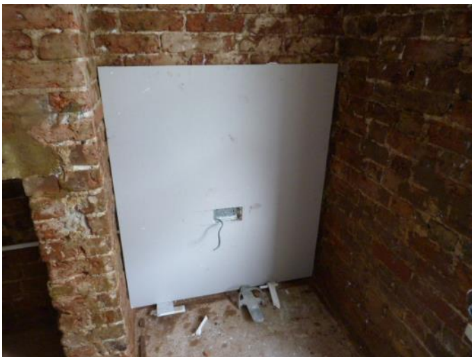
Dryshield applied behind the electrical socket backplate.
