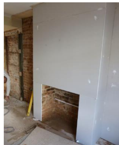
Plasterboard in one section around fireplace.
