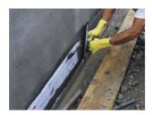
**2.** Immediately place the VANDEX CONSTRUCTION JOINT TAPE in the freshly applied VANDEX BB 75 E coat. Then, embed both fabric edges in the VANDEX BB 75 E
