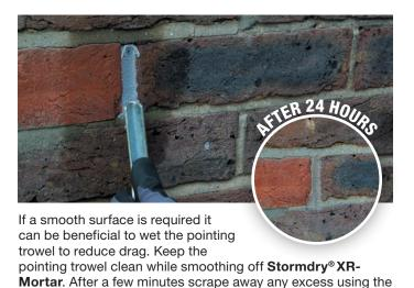
Stormdry® XR-Mortar cures by evaporation of moisture. In cold and damp conditions this drying process can be slowed, especially when applied in thick layers. For thick applications it may be necessary to apply the mortar in two layers to achieve an even cure. When applying the second coat push the mortar into the first coat for a good bond.
