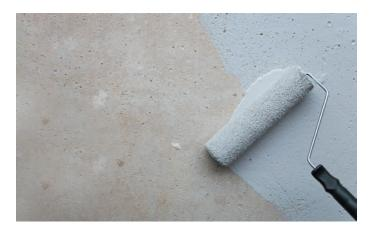
Where **Drybase® ECS Epoxy Floor Coating** is being used to provide a decorative surface it should be applied by skilled operatives familiar with the application of epoxy coatings to a high decorative standard. To ensure an even finish, special attention should be paid to:
