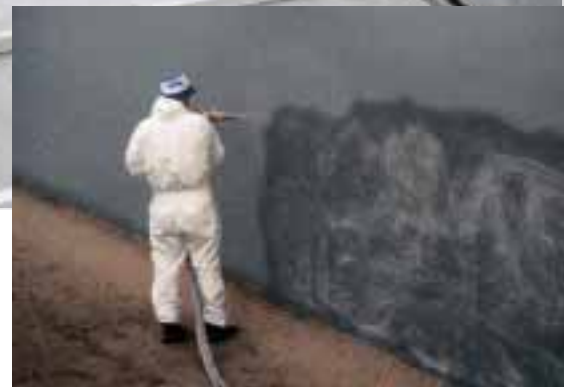
Spray application VANDEX POLYZEM Z
