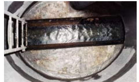
6. The refurbished manhole
