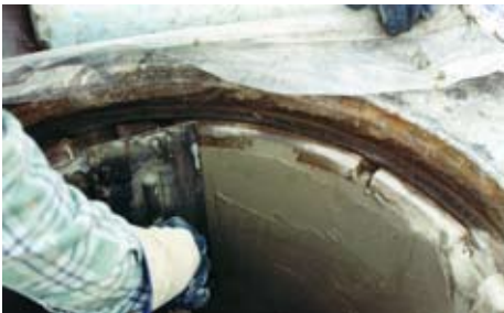
4. Reprofilling the top of the manhole with VANDEX RAPID S
