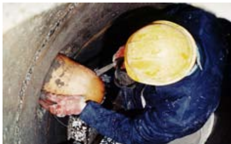
2. Plugging of damaged pipe inlets and joints
