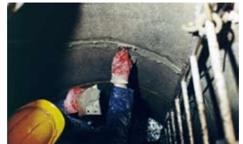
3. Sealing leaking joints with VANDEX RAPID M
