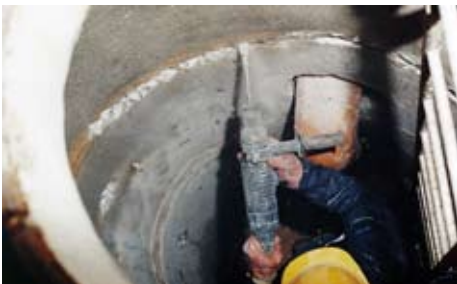
1. Pretreatment of cracks and joints
