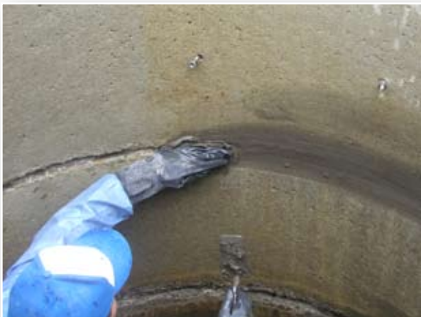
Sealing leaking joints
