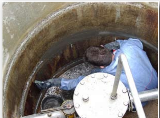
Sealing of leaking points
