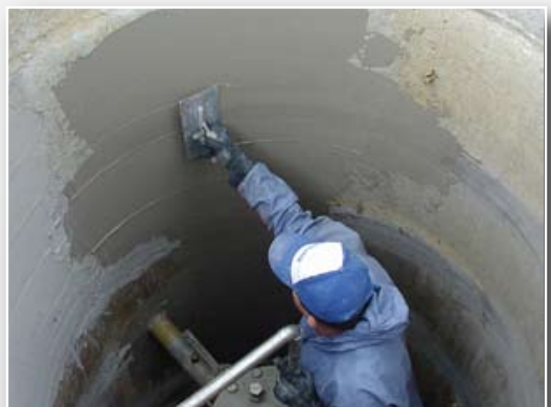
Waterproofing the surface
