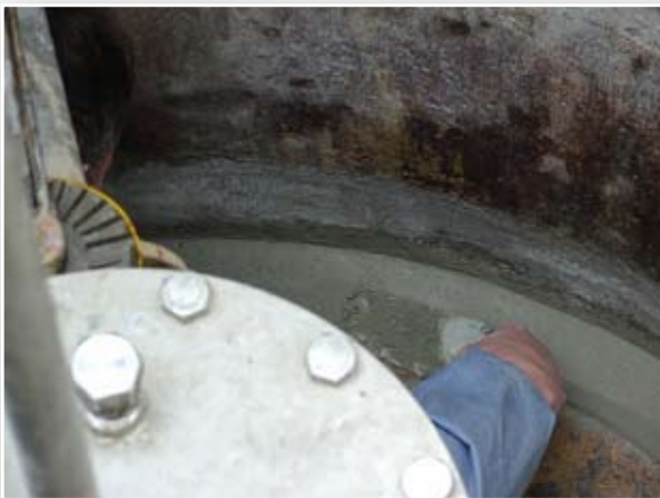
Applying a covered fillet at wall / floor junction
