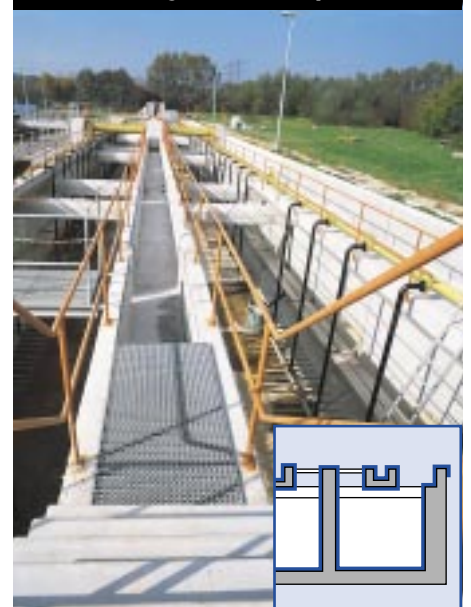
Sewage treatment plant
