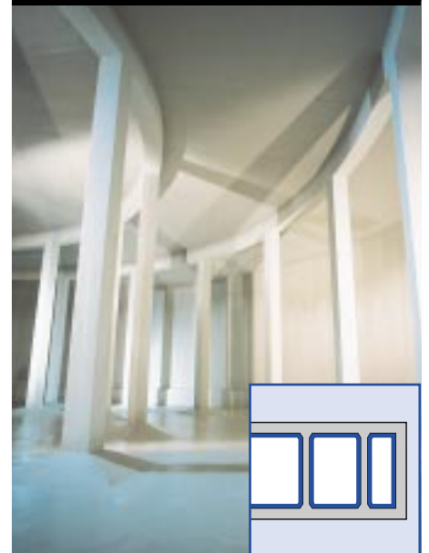
Drinking water reservoirs
