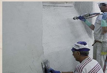
**Refurbishment of older structures:** Put an end to moisture that rises through capillary action from rising damp, moisture absorption from hygroscopy, and condensation from atmospheric moisture – Vandex saves older structures.
