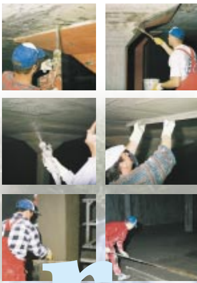
VANDEX CEDLINE MORTAR and VANDEX CEDLINE TOP GREY. Application mechanically and by hand.
