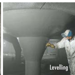
Spraying levelling mortar
