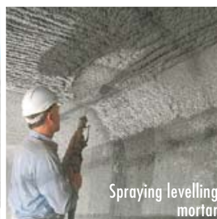
Substrate preparation
