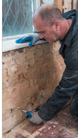
Installation of Dryrod® Damp-Proofing Rods .
