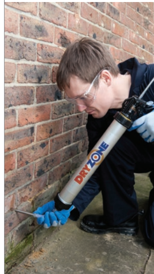
Injecting a new damp-proof course using Dryzone® Damp-Proofing Cream .
