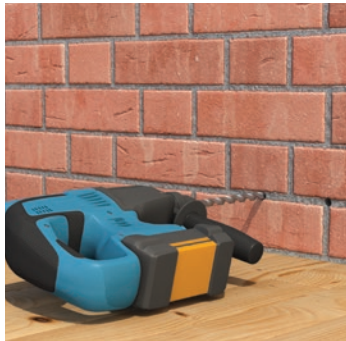
Drill holes at 120 mm intervals.
