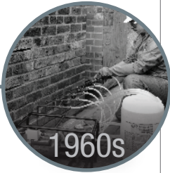
High pressure liquid injection
