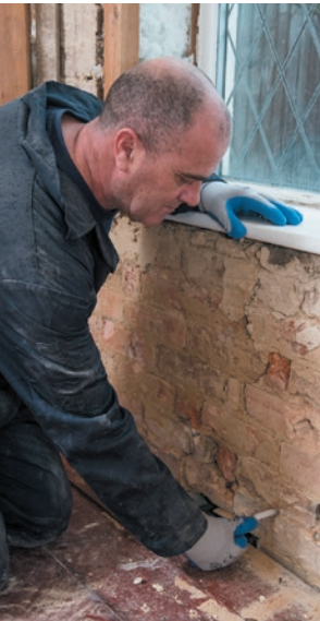
Installation of Dryrod® Damp-Proofing Rods.
