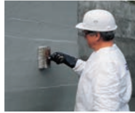
VANDEX Super applied as a slurry
