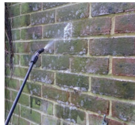
Pump sprayer and spray to wall
