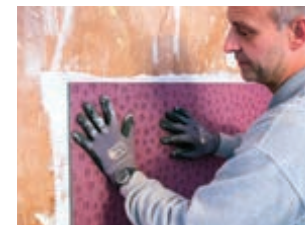
The same wall following application of Ultratherm
