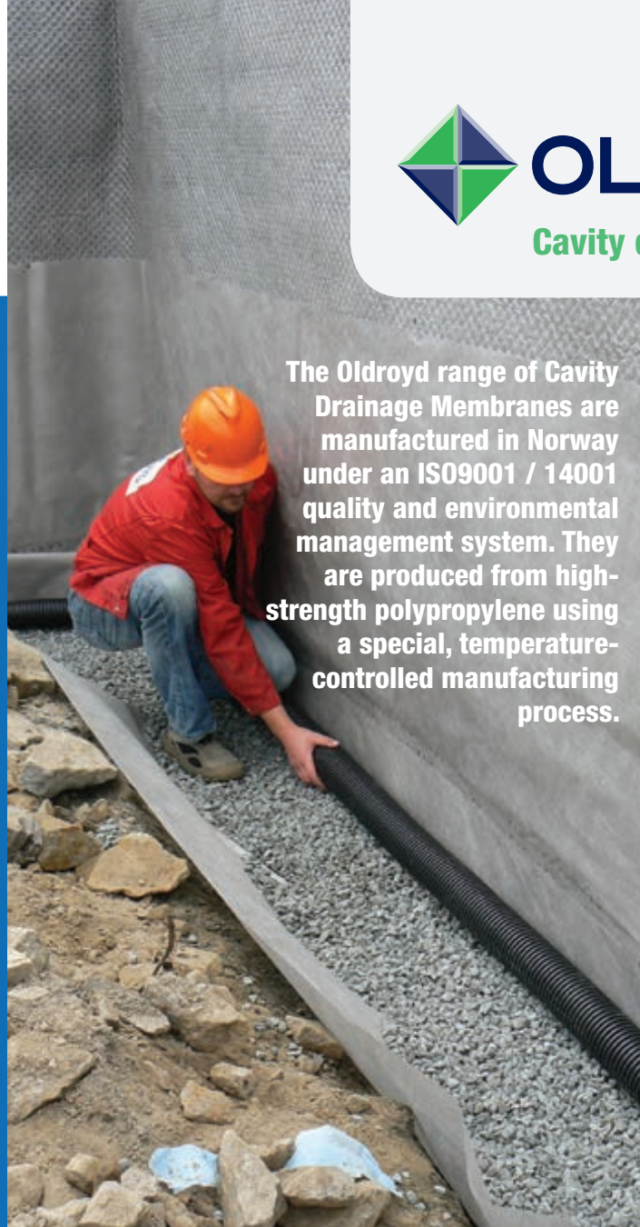
External Basement Waterproofing
