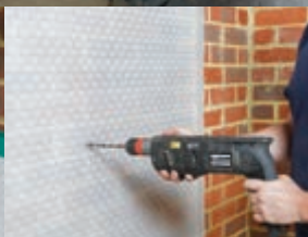
Drill holes for Oldroyd Brick Plugs
