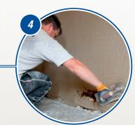
Apply the Plaster Coat Once the rough coat has become firm, apply the plaster again with a thickness of at least 15 – 20 mm.
