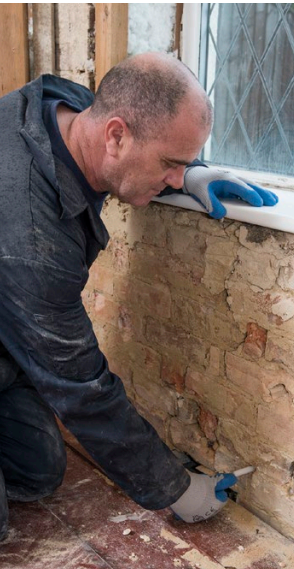
Installation of Dryrod Damp-Proofing Rods.
