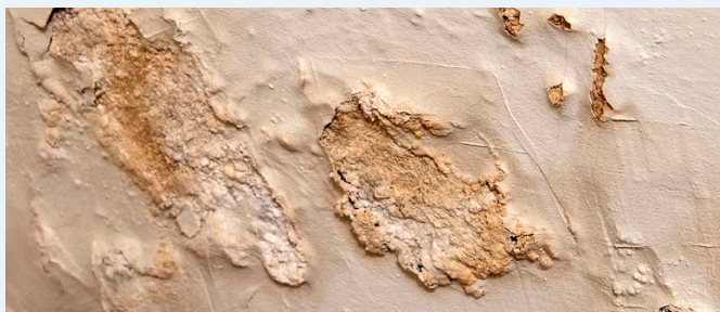
Hygroscopic salt contamination – Heavily salt-contaminated plaster will always need to be replaced – irrespective of which damp-proofing system is used.
