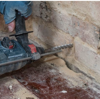
Drill holes at 120 mm intervals.
