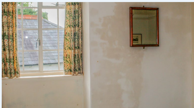
Hygroscopic damp – In this case it has not been caused by rising damp, but by hygroscopic salts in a chimney breast caused by the burning of coal.
