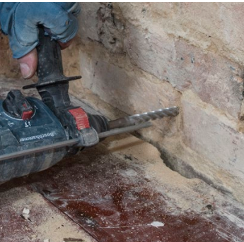
Drill holes at 120 mm intervals.
