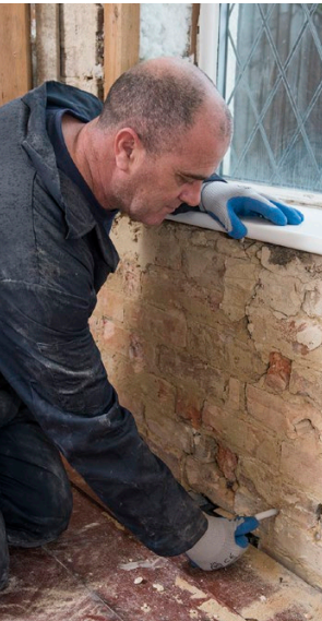
Installation of Dryrod Damp-Proofing Rods.
