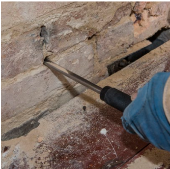
Clear the drill holes using the Hole Clearing Tool.
