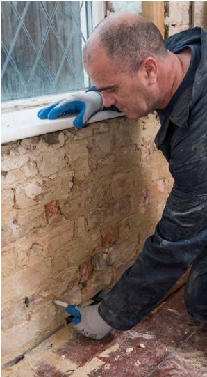
Installation of Dryrod Damp-Proofing Rods .
