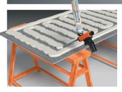
Lay the **Stormdry® EP-Board** on the ground with the dark-grey aerogel blanket facing up. Apply **Stormdry® EP-Board Adhesive** in a continuous line inset approximately 30 mm from the edge of the board until the entire perimeter has been covered. Infill the remainder of the board with the adhesive in a single, wide zig-zag pattern.
