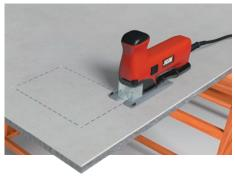
In order to completely cover a wall, it will most likely be necessary to cut some **Stormdry® EP-Board** down to size. Cutting should be carried out outside or in a well-ventilated area with an appropriate dust sheet. Always wear the correct PPE equipment including gloves, goggles and a dust mask. Cutting should be done using either a jigsaw or a mechanical saw. Cuts should always be made from the light grey Magnesium Oxide face of the board.
