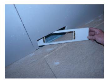
Secure the frame in this position by screwing through the plasterboard using two (4 x 25mm) screws on each side of the hole.
