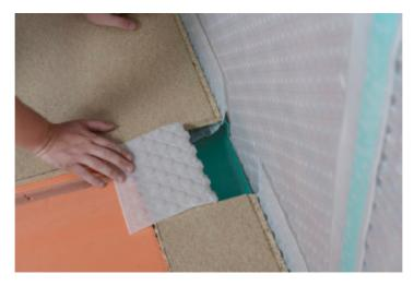
Remove any tapes from the floor/wall join and fold back the floor membrane giving you direct access to the Aquadrain. The lid of the Aquadrain can now be cut with the Multitool to allow access into the channel.
