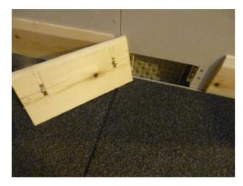
Snap the skirting into position and fit remainder of skirting boards. The skirting panel can be removed through the careful use of a flat head screwdriver or knife.
