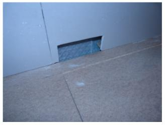
Insert the Access Point frame through the hole in the plasterboard and attach it so that the position the Access Point is 10mm off of the floor.
