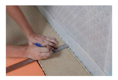
Keep the "cut out" section to insert back in the aperture to protect the floor membrane during dry lining works. If a screed is to be installed, then a screed box must be positioned against the wall prior to the pour in order to achieve the same access.
