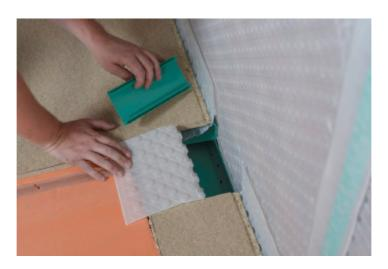
When returning the floor membrane to its original position over the Aquadrain the edges must be sealed with Oldroyd Overseal tape. If there are any problems with folding back the floor membrane or if it becomes damaged then simply cut and remove it. A piece of Oldroyd Overseal tape can be used over the aperture in the membrane to seal it.
