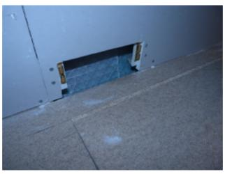
With the male fittings in the ball catches, measure from floor to centre of male fitting. This measurement should be 50mm. It is important to have the male fittings at the mid-height of the skirting board to ensure a secure fit.
