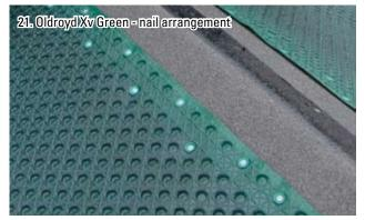
Fixings should be staggered with a minimum spacing of 400mm at pitches below 20°, and 200mm for over  $20^\circ$  pitch.
