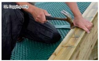
To stop water getting underneath the Oldroyd Xv Green membrane around the edge of the roof, a capping strip must be installed along the perimeter upstand.
