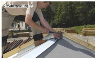
Ensure the roofing felt overlaps at the apex (ridge).
