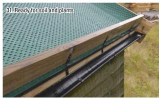
The construction, waterproofing and drainage is now ready for the installation of the soil and plants.
