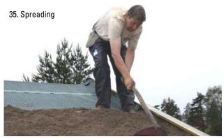
The soil should be spread evenly to a suitable depth for the plants. This will vary according to the chosen plant, check with your supplier.
