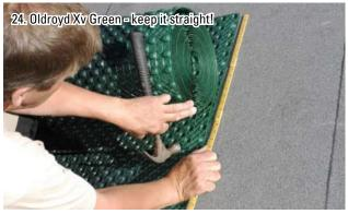
When working up the roof, ensure that the new layer remains parallel to the previous layer.
