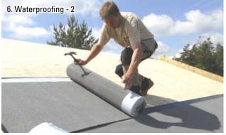
Working up the roof, roll out the next roll of roofing felt and tack into position. With temperatures less than around 0°C, warm the overlapping adhesive with warm air. It is inadvisable to use a naked flame.
