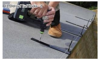
Turf hooks should be installed in line with the rafters, at spacings no greater than 500mm.
