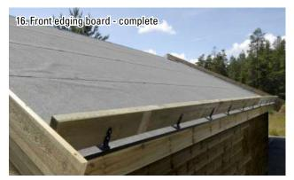
The completed board runs along the full length of the roof
