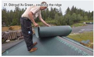
The final roll should be applied centrally over the ridge of the roof. Ensure overlaps are greater than the minimum requirement for pitch of roof (see step 23).
