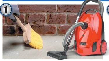
Before application, sweep the area to remove any loose material, then vacuum thoroughly. Dampening the area will help 'wetting out', but do not leave any standing water. Unsound surfaces will need to be primed before application.
