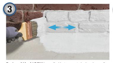
**Drybase® Liquid DPM** is applied in two coats by brush or roller. Apply the first coat, moving in one plane, back and forth. Allow the first coat to become touch dry – usually 1 hour.
