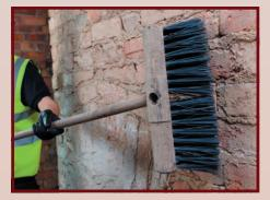
Before applying **Drybase**® **Flex Membrane** below ground, consider any pipes, electrical outlets, anchoring points, corners and overlaps – see 'Detailing' section. Section 8.1.3 in BS 8102 states that continuity of the waterproofing system be maintained and penetrations through walls and floors should be avoided. The structural integrity of the slab should be considered before any waterproofing commences.
