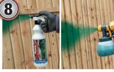
When spraying **Roxil® PC**, hold the nozzle 15-30 cm from the wood surface and apply in 2-3 even coats for the desired finish. Keep a brush handy to blend in any over-saturated areas, runs or streaks. Wait until touchdry between coats.
