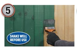
**Roxil® PC** can be applied by large brush. Use a smaller brush for application around details such as shed windows. Apply in 2 – 3 even coats to achieve the desired colour, brushing along the grain. Wait until touch-dry between coats.
