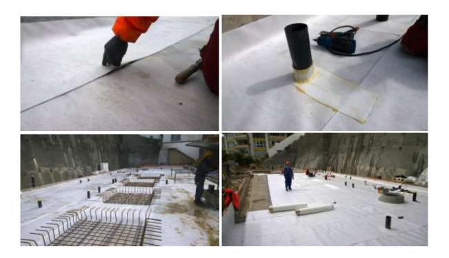
**Note:** DualProof is designed for use with structural reinforced concrete. The concrete should be designed by a Structural Engineer to EN 1992. Please ensure that the concrete is placed and cured correctly, and that all non-movement construction joints are detailed with CEMflex Active Waterstop.
