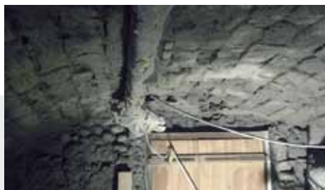
4 First layer; VANDEX UNI MORTAR 1
