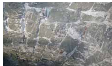
3 Damaged plaster removed
