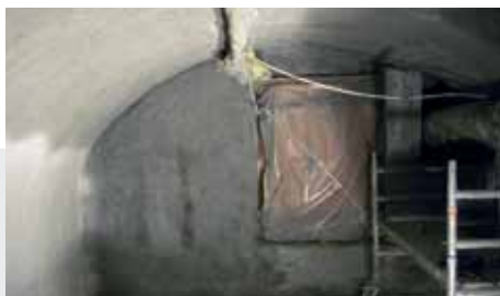
5 Second layer; refurbishment plaster
