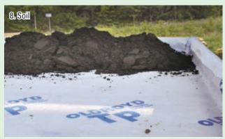
The roof soil or substrate is then loaded on to the roof by placing it directly on top of the filter fleece.
