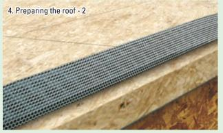
Perimeter upstands will be required to retain the soil and plants. Ensure the draining edge is perforated or a gap is created for free drainage of excess water off the roof.
