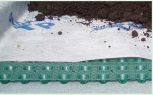
Good quality exterior grade flat roof waterproofing membrane, root barrier (if not provided by the waterproofing membrane), Oldroyd Xv20 GreenXtra drainage membrane and Oldroyd Tp filter fleece.
