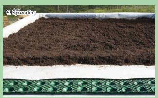
The soil or substrate should be spread evenly to a suitable depth for the plants. This will vary according to the chosen plants (check with your supplier).
