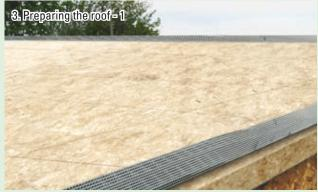
A roof is typically constructed from a timber or concrete deck, with a minimum 1° pitch to prevent ponding. Ensure it is strong enough to take saturated weight of soil and plants (check with supplier).
