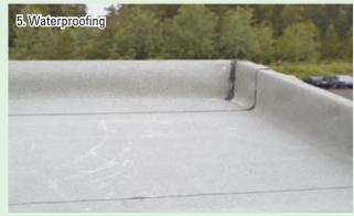
The roof should be waterproofed with a good quality exterior grade flat roof waterproofing membrane, and any penetrations should be waterproofed accordingly. It is recommended that waterproofing is done by an experienced contractor. Guttering should now be installed if required.
