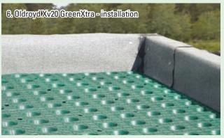
If the waterproofing layer is not a root barrier, then a physical root barrier should be installed on top of it. The Oldroyd Xv20 GreenXtra sheets are loose laid on top of the waterproofing/root barrier. Note that the sheets will be held in place by the weight of the soil and plants.
