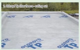
The Oldroyd Tp filter fleece is rolled out over the drainage membrane and returned up around soil to prevent any soil loss. A 300mm gravel border is recommended to provide ballast, prevent soil erosion at edges and act as a fire break.
